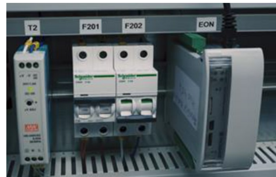
Figure 72 – Typical control cabinet (left) and typical E.ON Energy Manager mounting (right)
