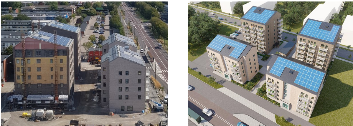
Figure 12: The four multifamily homes during their construction
